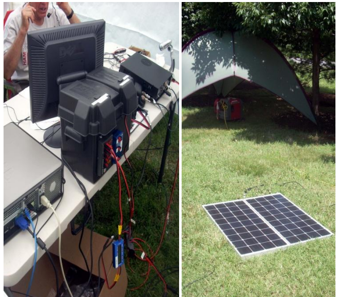
Battery, generator and solar power supplied the energy required to operate Field Day totally off the grid.
