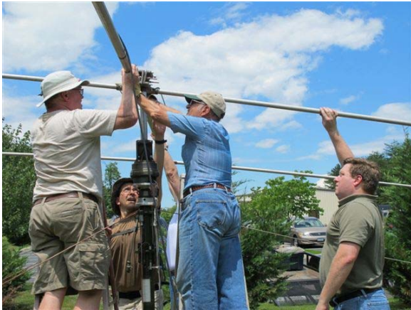
Jim K4CGY, Mike KJ4MFN, Wes K4WLE and Dave K4DND get the 20M beam on the rotator
